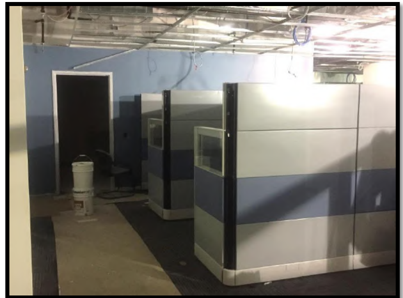
Current work on 2 nd floor
